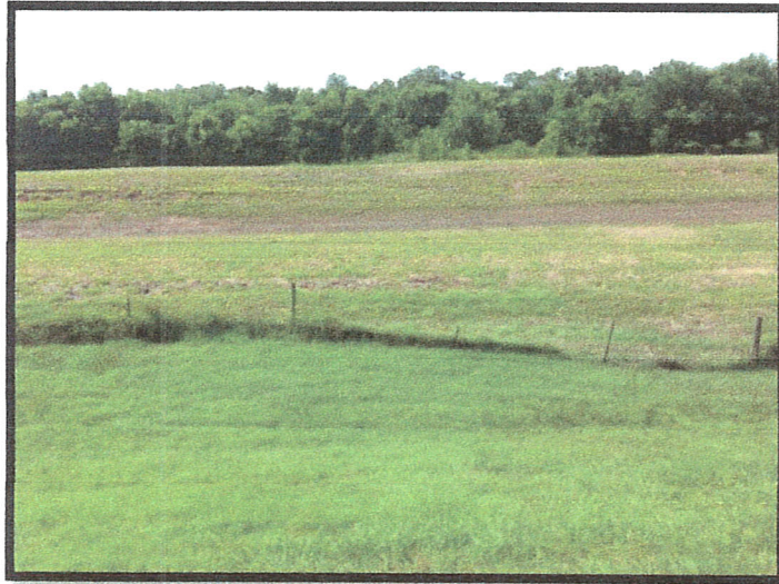
Hog Fencing repairs
