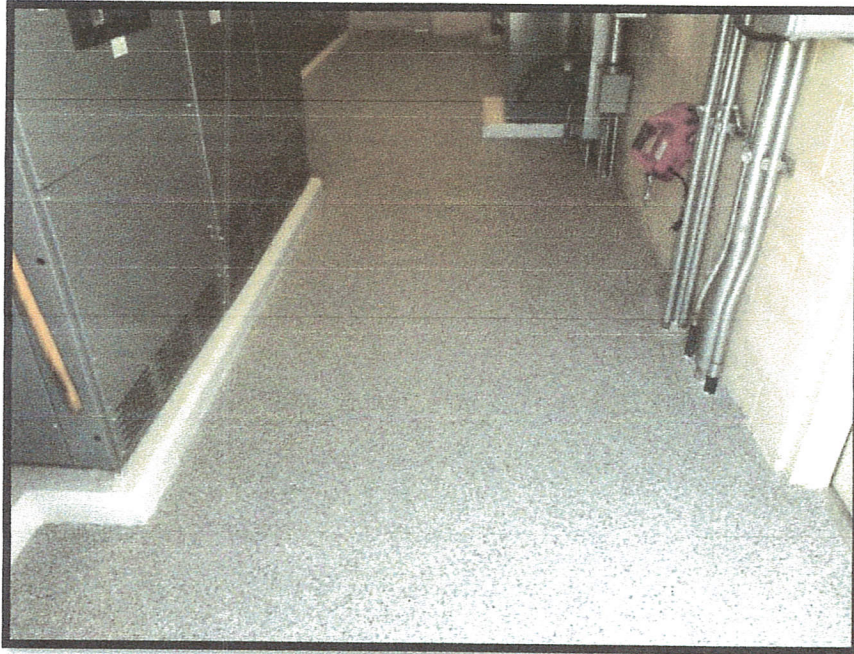
Epoxy Floor Install
